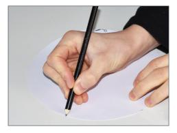
1. Once you have a suitable position for the antenna, cut out the supplied template. Use to mark the 25mm centre hole position and mark the outside of the antenna.
